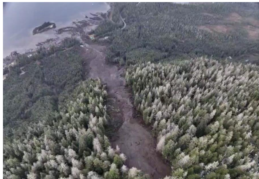
Landslide outside Wrangell in Southeast Alaska Photo credit: Alaska Department of Transportation and Public Facilities
